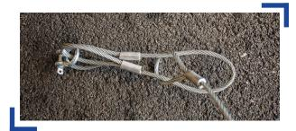
Run clevis back through the small cable and pull tight.
