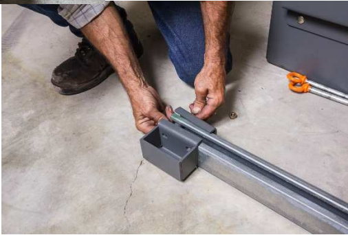
1/2" Bolts shown installed in Roller Assemblies
