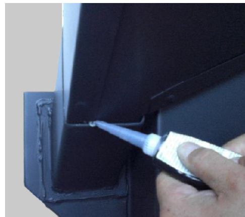
Fill the entire void.
