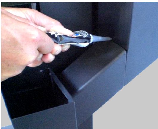
Apply silicone around all four edges.
