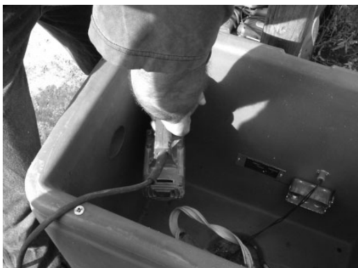
Illustration 6 - Transfer & Drilling Holes
