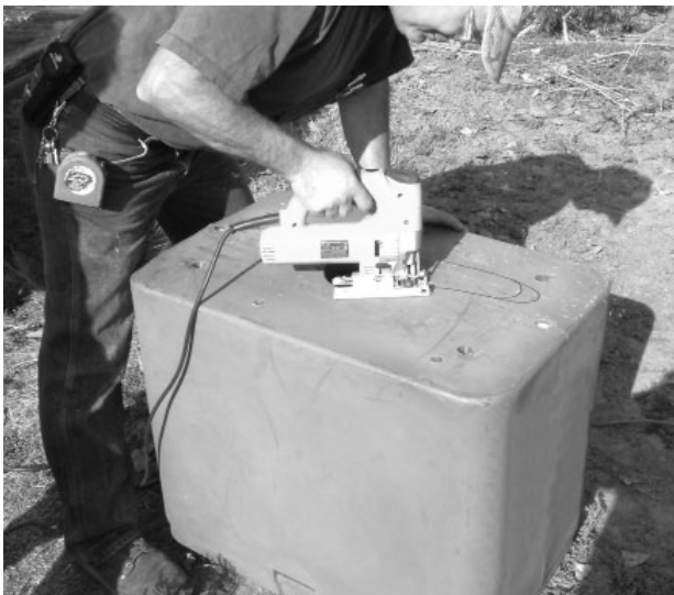
Illustration #2 - Enlarge Hole As Needed
