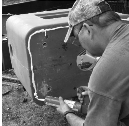
Illustration 7 - Caulking Bottom
