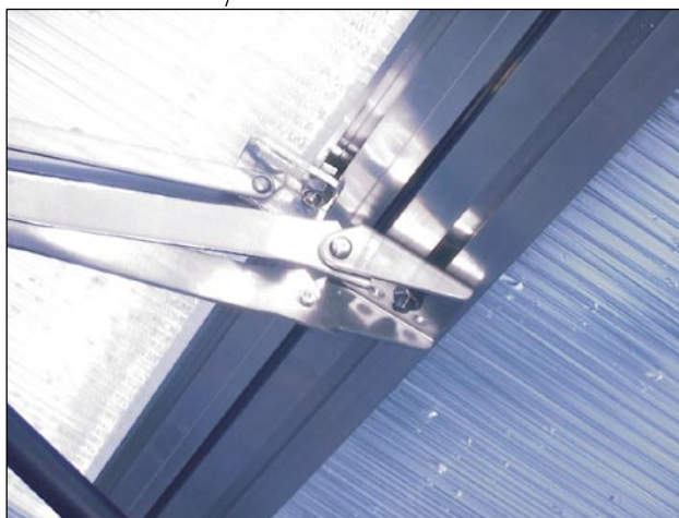
automatic roof window opener
