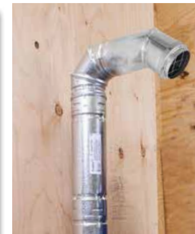
10. Attach horizontal cap to the top elbow.
