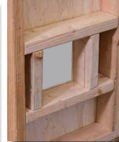
2. Cut and frame wall penetration.
