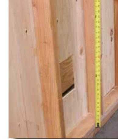
1. Locate appliance and penetration through wall.
