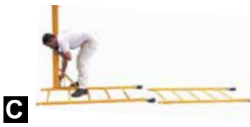
C Attach one Side Brace to top of Side Frame, then secure it with the Lock Pin.
