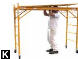
K Insert Wood Platform, firmly position it on top of both Side Braces.
