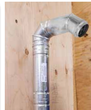
10. Attach horizontal cap to the top elbow.
