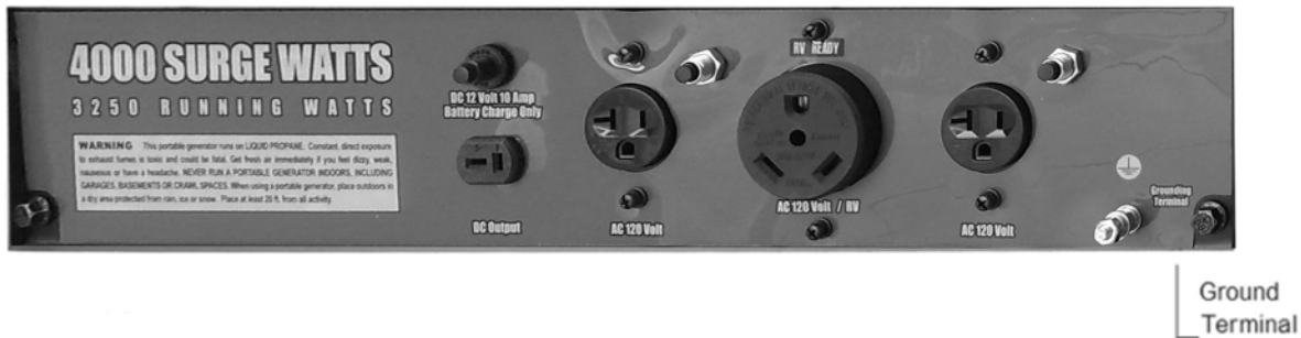
Figure 3 - Attaching the Grounding Wire to this Generator
